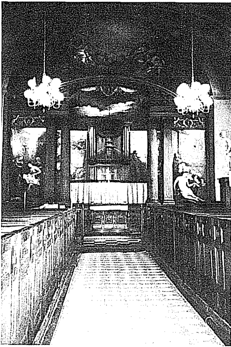
Interior view—Church of St. Lawrence, Whitchurch, Canons Park.
